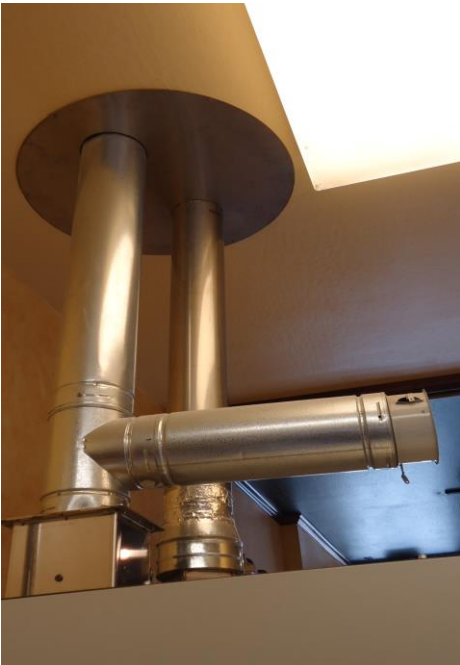
Example of gas exhaust with barometric damper. (See schematics for alternative layouts.)
